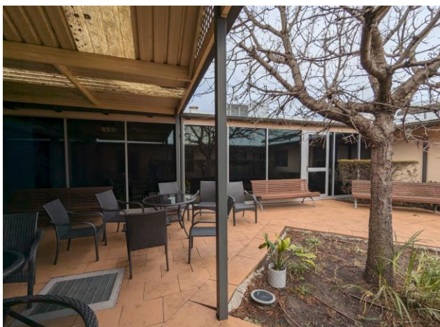
Picture 1 Existing Courtyard
